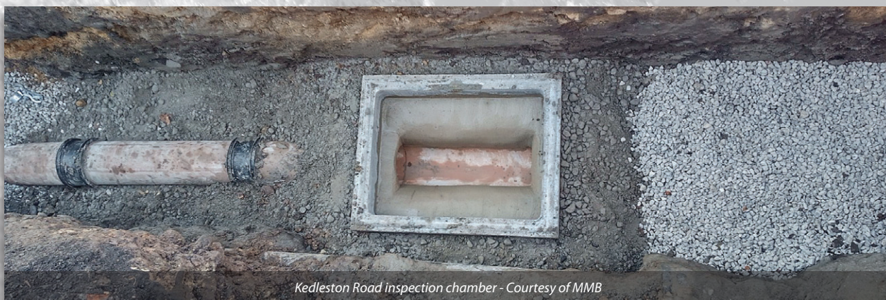
Membrane-lined bioretention trench with perforated pipe and granular bedding Courtesy of MMB
