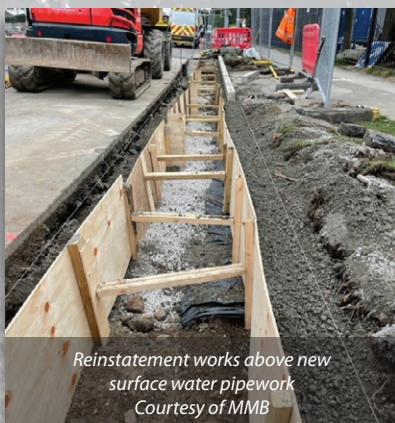
Membrane-lined bioretention trench with perforated pipe and granular bedding Courtesy of MMB
