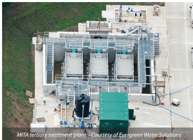
External mounted backwash pumps Courtesy of Evergreen Water Solutions
