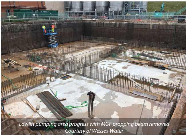
Excavated lowlift pumping area (LPA) with single concrete pour for base in progress - Courtesy of Wessex Water
