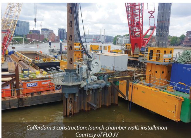
Cofferdam 3 construction: launch chamber sheet piles installation Courtesy of FLO JV
