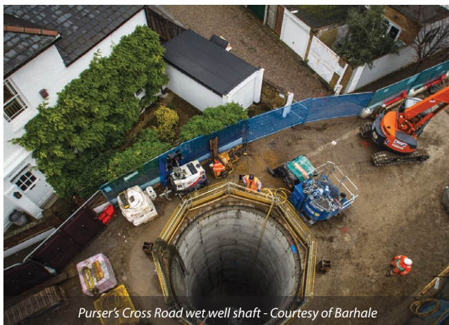
Purser's Cross Road shaft sinking - Courtesy of Barhale
