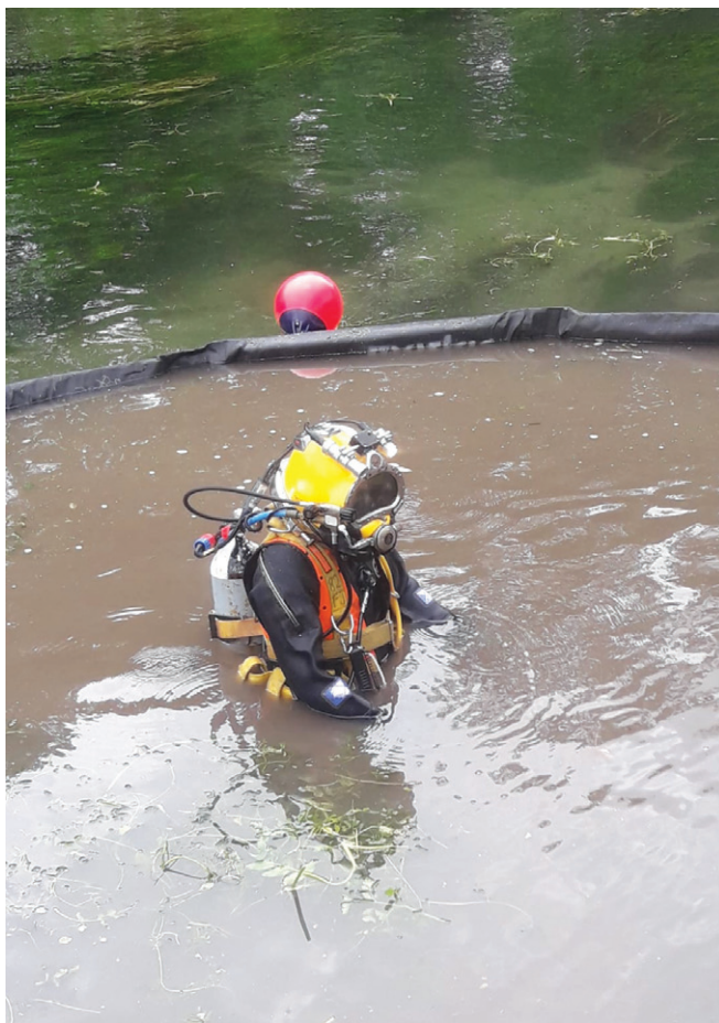
Silt curtain in place and dive works underway - Courtesy of BTU Utilities
