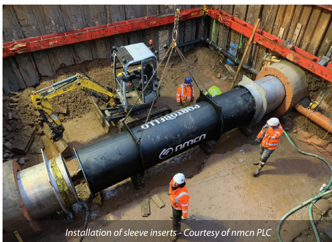
Bespoke sleeve inserts and flume for brick egg sewer - Courtesy of nmcn PLC
