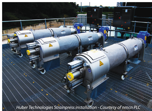
Automated Strainpress feed installation - Courtesy of nmcn PLC
