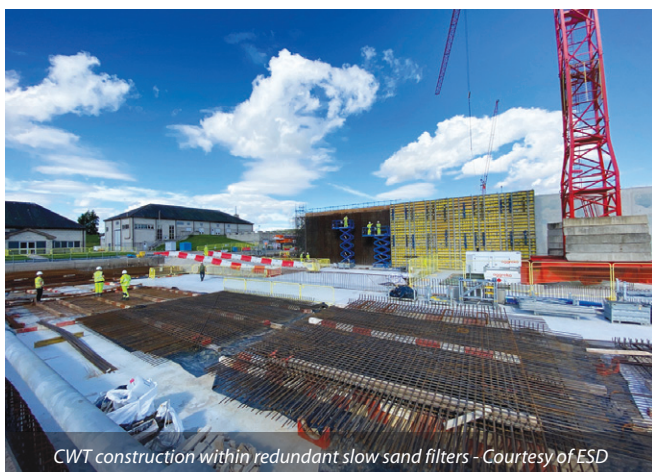
Enabling works within redundant slow sand filters - Courtesy of ESD
