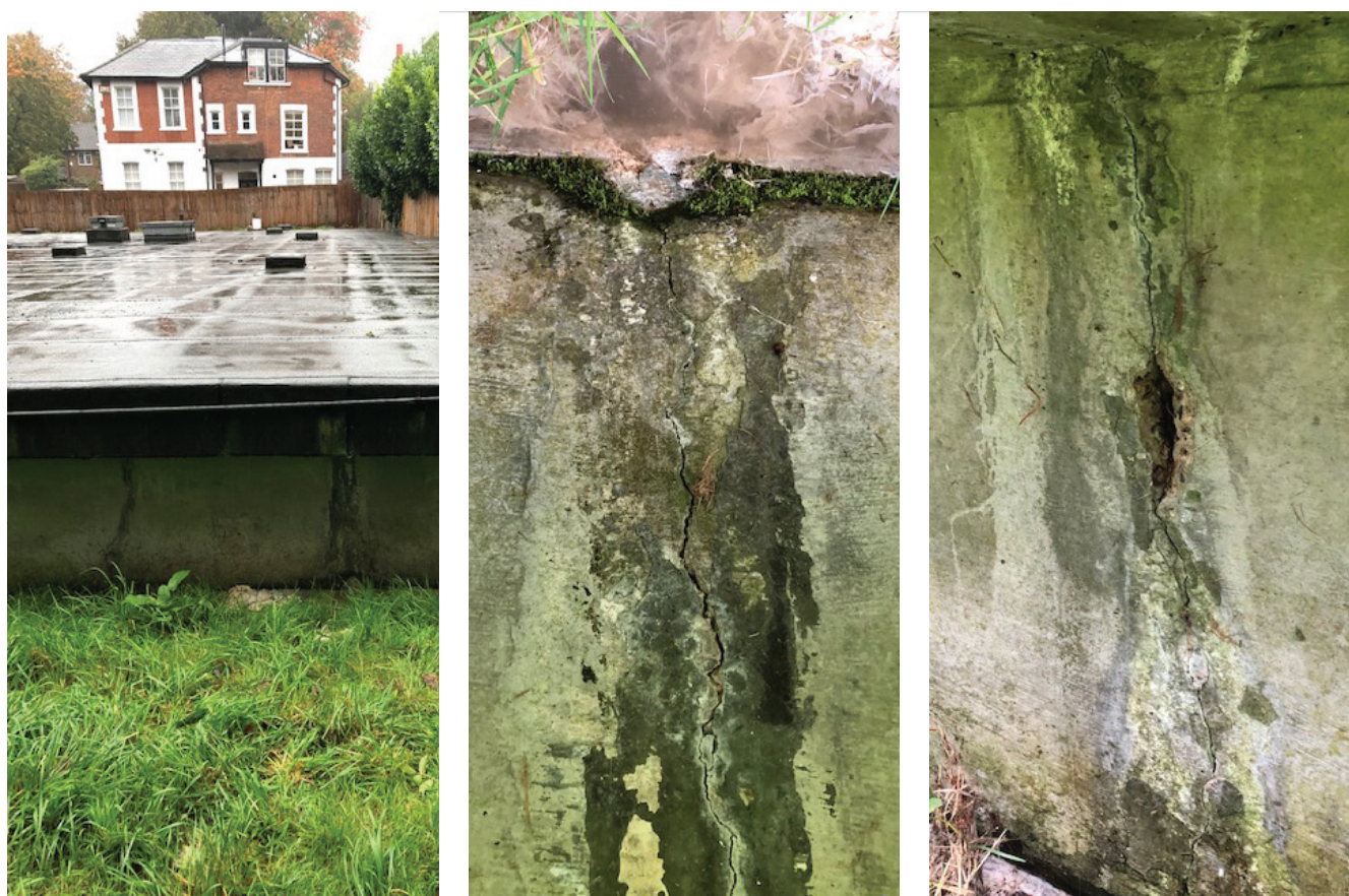
Photographs of leaking cracks observed in November 2019 - Courtesy of South East Water
