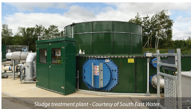
Clean backwash tank and GAC filter - Courtesy of South East Water
