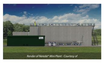
Nereda Package Plants have been developed to provide a factory built, competitive, sustainable, lowest whole life cost solution. In addition to meeting the P removal requirements, the package plants have also been designed to meet high standards of nitrogen removal and Nereda technology is well proven for achieving treated water ammonia consents down to 1 mg/l and Total N consents well below 10 mg/l.
