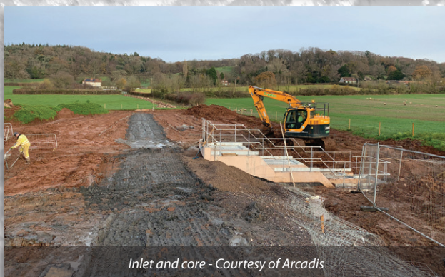
Cut-off clay core construction - Courtesy of Arcadis
