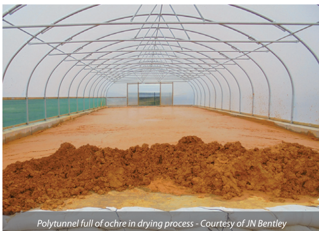
New sludge drying bed following first de-sludge - Courtesy of JN Bentley
