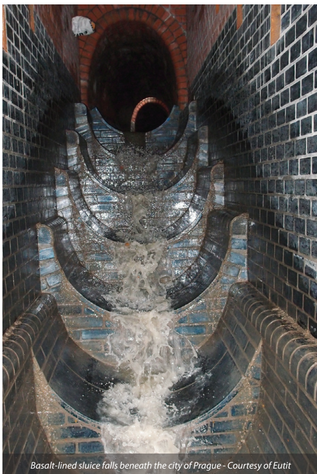
Repaired section of Prague's sewer system - Courtesy of Eutit
