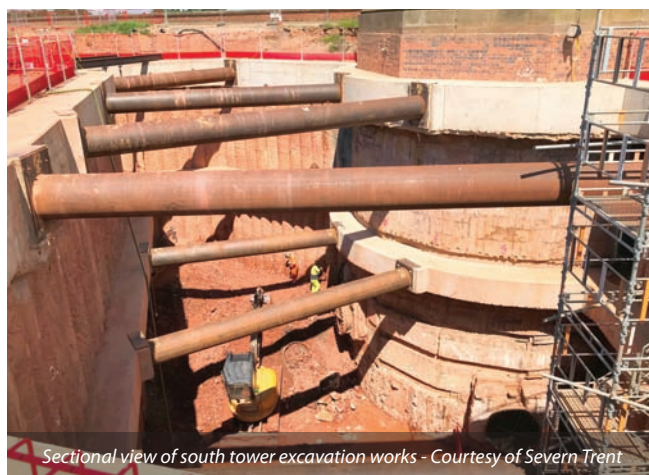
Excavation works for south tower pipework connection Courtesy of Severn Trent
