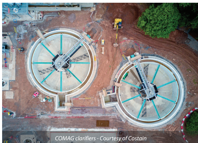
Tertiary treatment process (COMAG) - Courtesy of Costain
