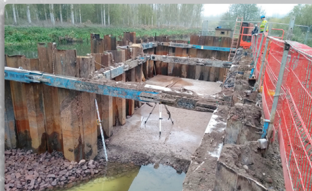
Blinding base - Courtesy of nmcn PLC
