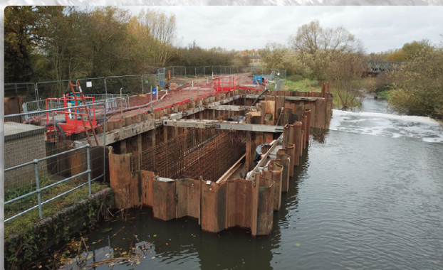
Extensive cofferdam - Courtesy of nmcn PLC
