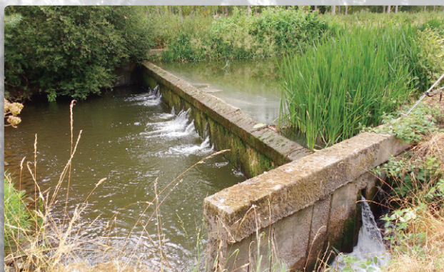
The original weir was a barrier to fish passage - Courtesy of nmcn PLC
