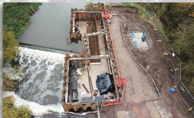
Construction underway within the cofferdam - Courtesy of nmcn PLC
