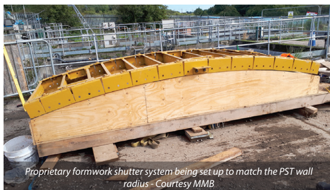
Temporary works for the PST sludge hopper - Courtesy of MMB
