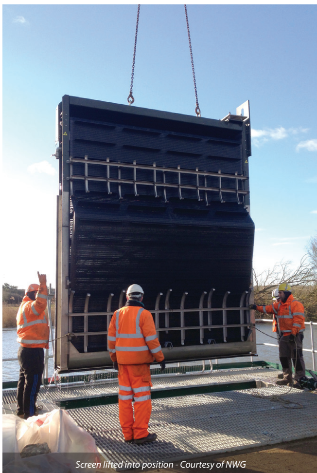
Screen positioned external to existing structure - Courtesy of NWG
