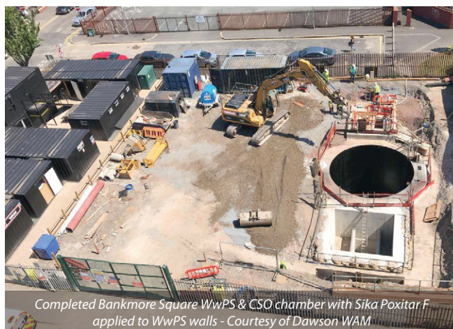
Circular secant piled Bankmore Square WwPS wet well with internal reinforced concrete liner wall - Courtesy of Dawson WAM
