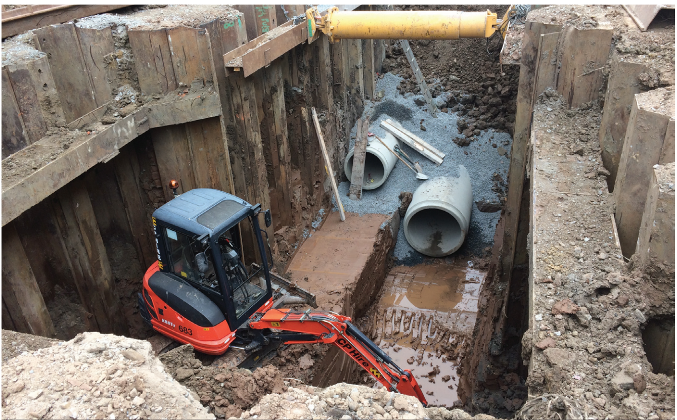
Sheet piled temporary works cofferdam for open-dig section of 1200mm combined sewer and 900mm overflow pipelines - Courtesy of Dawson WAM
