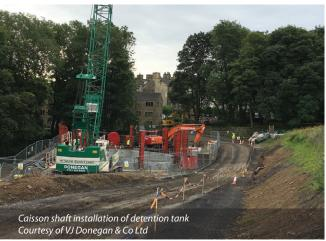
The use of online storage was investigated but the location and topography of the area meant that there was not the available space to store and gravitate flow back to the sewer network. There was, however, space in steeply sloping fields downhill of the properties. This meant that a storage solution would require a pumped return to the existing system.
