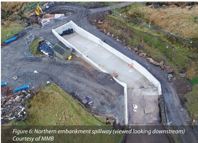
Figure 5: The existing northern embankment spillway Courtesy of MMB
