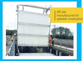
Integrated Fixed-film Activated Sludge (IFAS)
