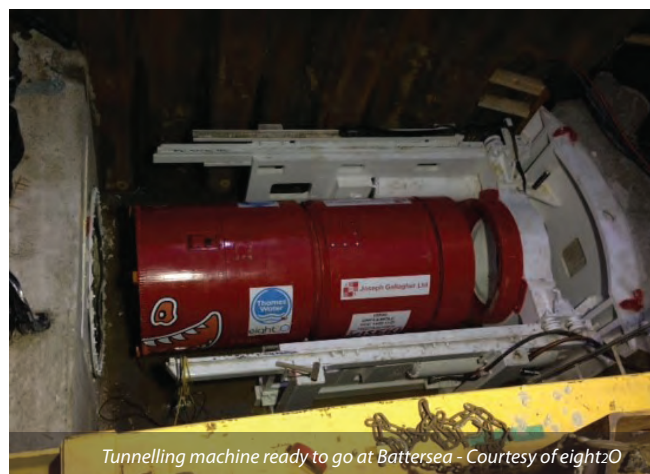
DN2400 Ridgistorm XL pipeline excavation - Courtesy of eight2O
