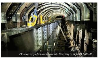
steel bridge needs to be fixed into place in case the sewer surcharges and requires evacuation.
