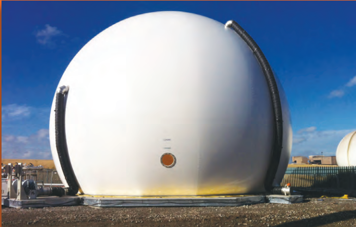
Double Membrane Gas Holder
