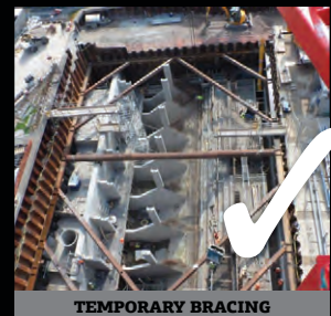
TEMPORARY BRACING
