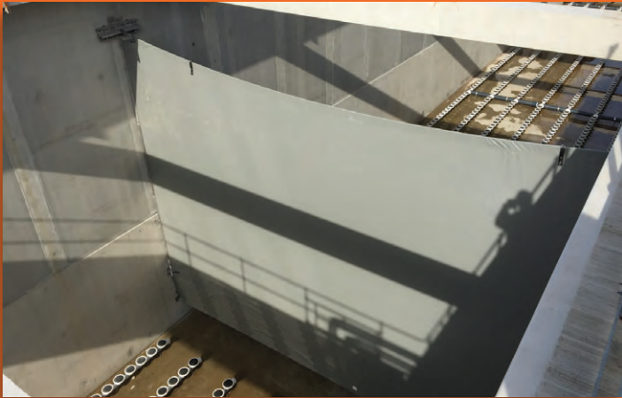
Structural custom fit Baffle Curtains for Process Tanks
