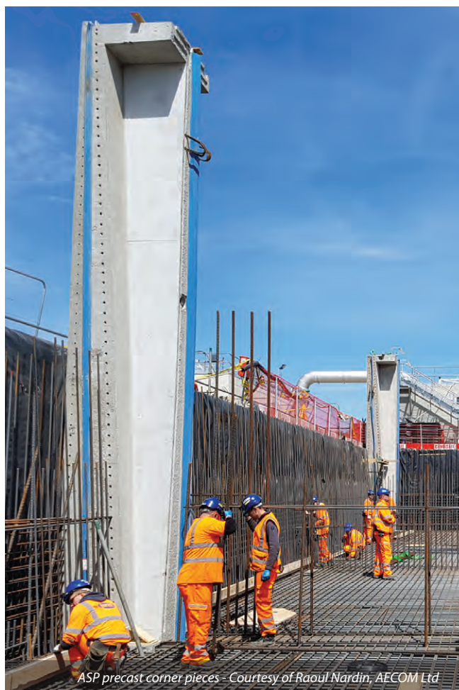
(Left) ASP precast middle unit and (right) precast corner unit showing complexity of reinforcement - Courtesy of AECOM Ltd
