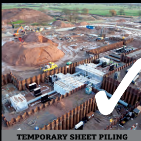
TEMPORARY SHEET PILING
