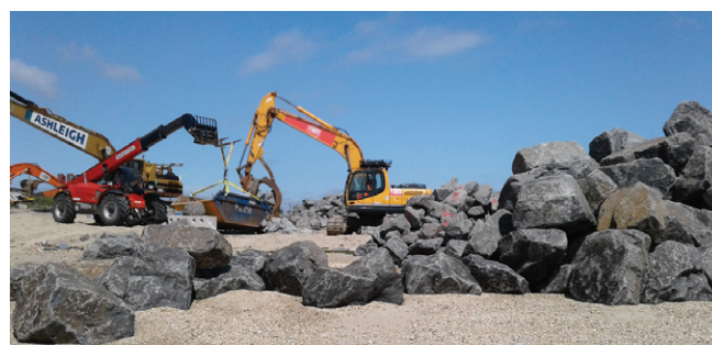
Machinery in full force to shift the rocks from the beach area to form the new sea defences - Courtesy of Southern Water
