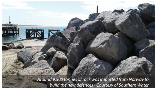
Rock armour is spread over 115m of beach area, adjacent to the historical Fort Cumberland - Courtesy of Southern Water
