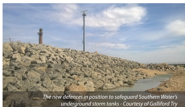
Around 9,500 tonnes of rock was imported from Norway to build the new defences - Courtesy of Southern Water
