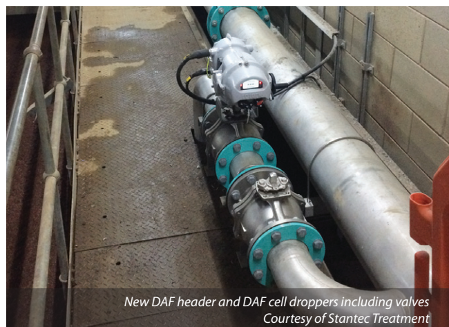
The new DAF Saturator pipework and valve assemblies and platform about the existing saturator vessels - Courtesy of Stantec Treatment
