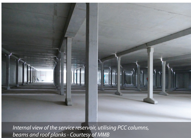
Using PCC units increases the quality through manufacturing in a controlled 'factory' environment - Courtesy of MMB
