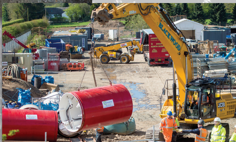
TBM installation lift SW/SNS Photography
