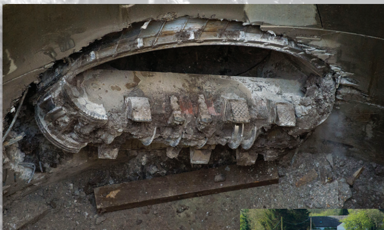
TBM breakthrough Courtesy of SW/SNS Photography
