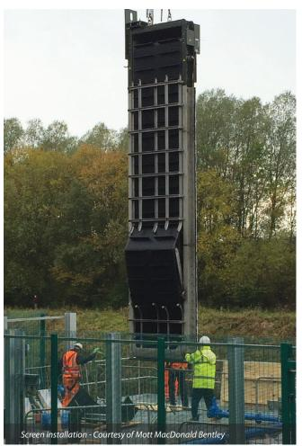
The preferred solution entailed installation of 4 (No.) environmental fish exclusion (EFE) screens within the flushing flow of the river. To accommodate this, a new steel support structure was installed on top of the existing concrete intake, constructed in 1975.
