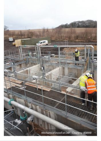
In addition to the PCC solution for the tertiary plant, Design for Manufacture and Assembly (DfMA) was used to reduce on-site construction and installation times, reduce working at height and improve site health and safety. For example, access metalwork was assembled in sections off-site, ready to be delivered, craned and fixed into position.
