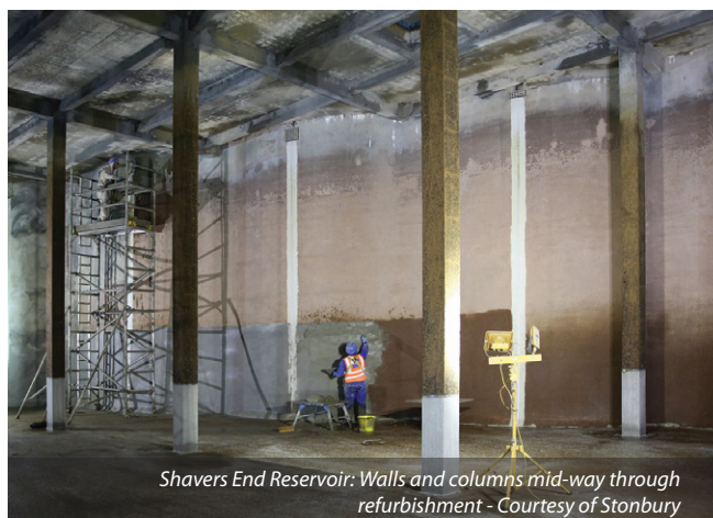
Shavers End Reservoir: Necessary checks being carried out to ensure that the correct application criteria as per the manufacturers IFU Courtesy of Stonbury
