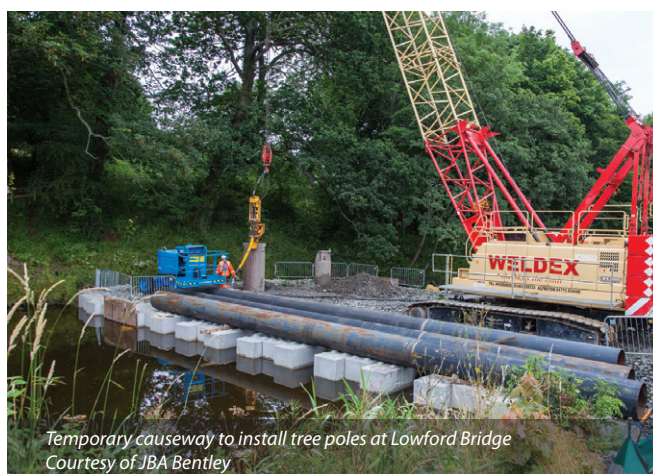
Temporary causeway to install tree poles at Lowford Bridge Courtesy of JBA Bentley
