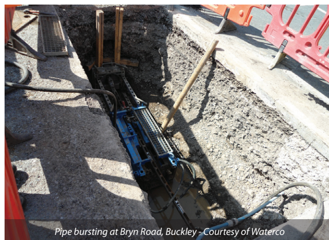
Pipe bursting at Bryn Road, Buckley - Courtesy of Waterco
