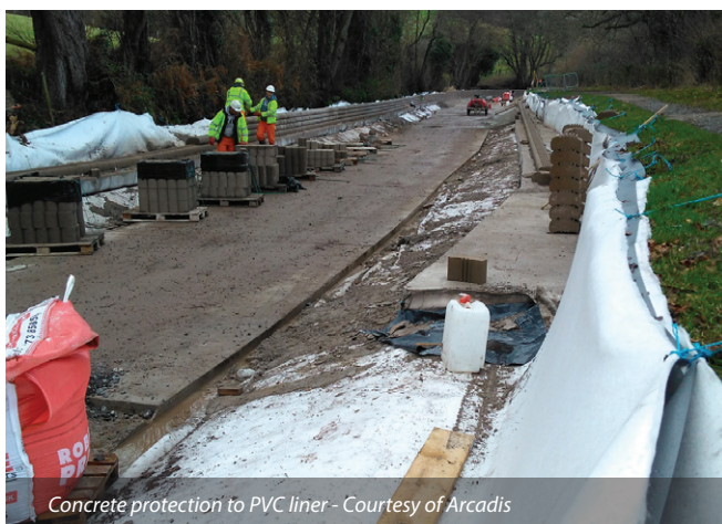
PVC liner installation on prepared canal bed - Courtesy of Arcadis
