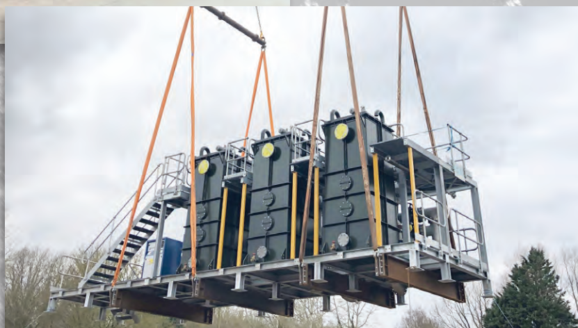
Tertiary treatment skid being craned into position - Courtesy of EPS
