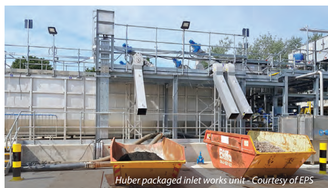
Packaged inlet works with integrated platforms - Courtesy of EPS
