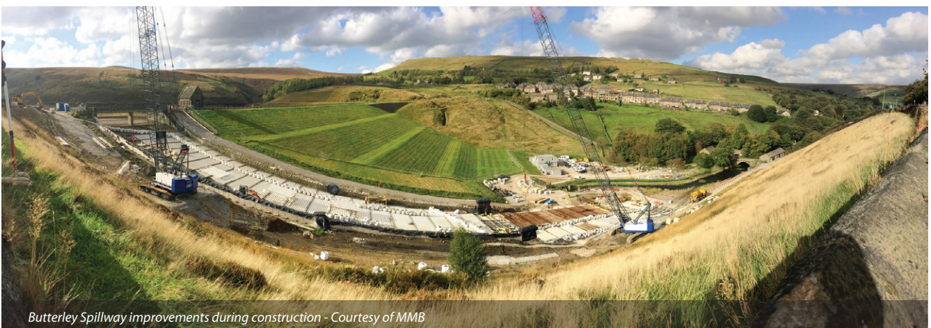
New concrete spillway and masonry walls - Courtesy of MMB
