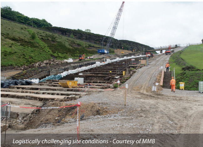
Bespoke formwork for in situ concrete - Courtesy of MMB
