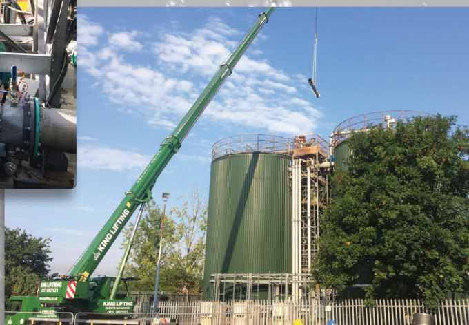
Lifting the gas draw-off pipe off the roof Courtesy of WECS
