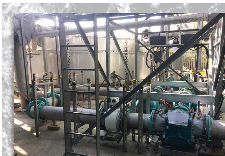
Duty/duty sludge transfer pumps for Tank 4 bypass in operation - Courtesy of WECS
