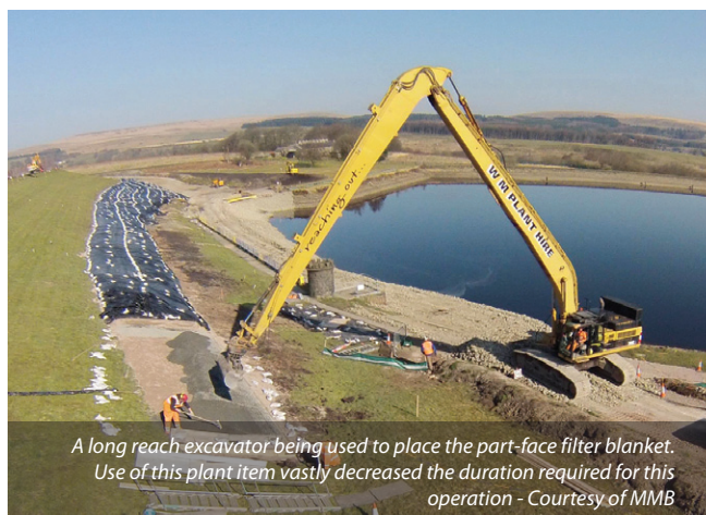
Filter material overlying drainage material (itself overlying filter material) within the part-face filter blanket. Formwork was used to ensure the correct layer thickness throughout - Courtesy of MMB
