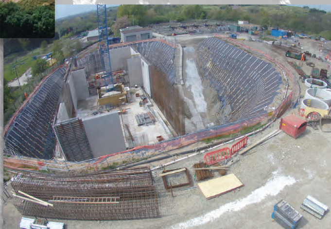
Royton WwTW - Detention tank Courtesy of United Utilities
