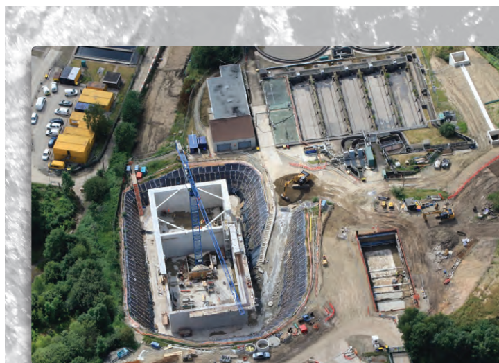
Royton WwTW - Detention tank, header tank (top right) and new CSO chamber (bottom right) - Courtesy of United Utilities
