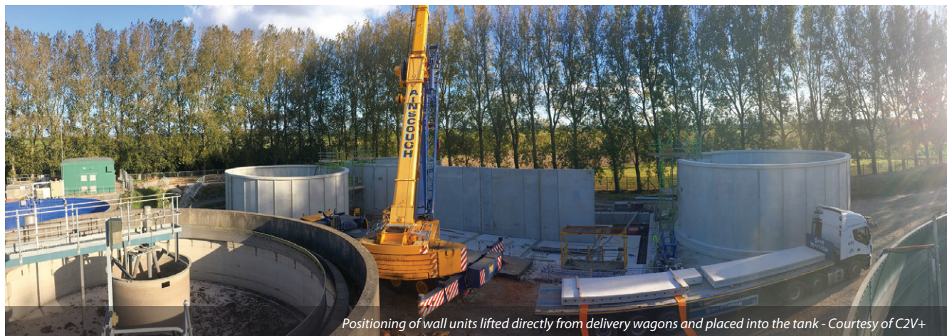
New process plant under construction - Courtesy of C2V+
