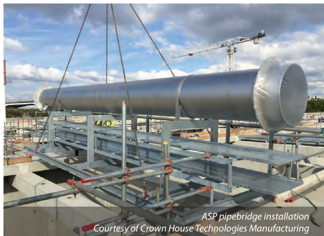
ASP pipebridge delivery Courtesy of Crown House Technologies Manufacturing
