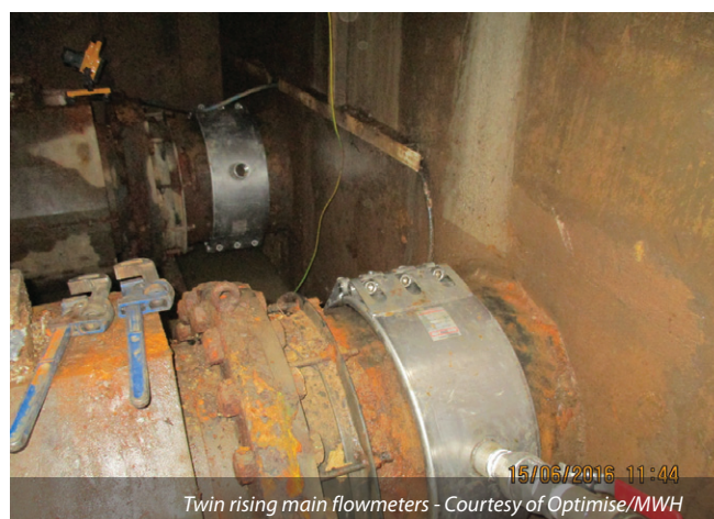
DSPS flowmeter - Courtesy of Optimise/MWH
