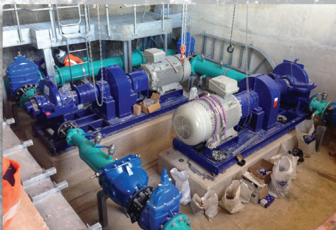
Figure 7: Whitefield C Water Booster Station pumps and manifold during installation - Courtesy of SMB
