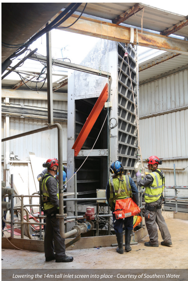
Lifting the inlet screens into position - Courtesy of Southern Water
