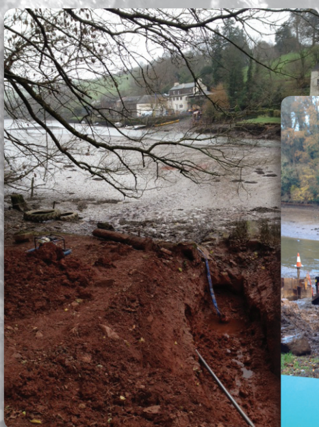
Successfully crossing the estuary with the directional drill rods - Courtesy of South West Water Delivery Alliance H50
