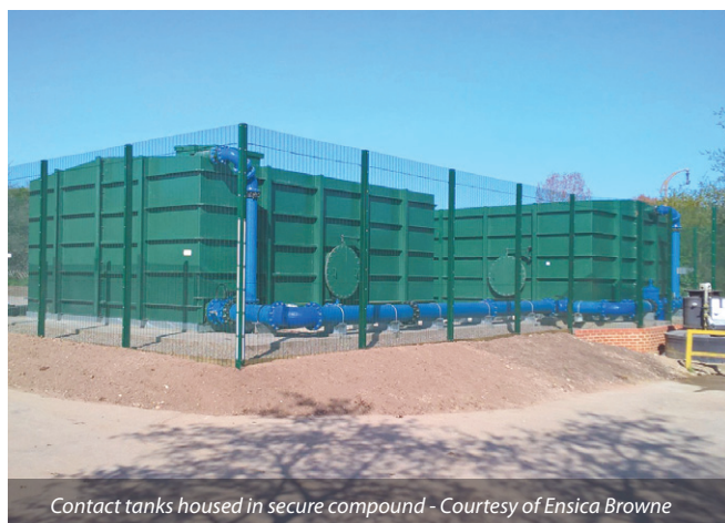
New contact tanks commissioned and in service Courtesy of Enisca Browne
