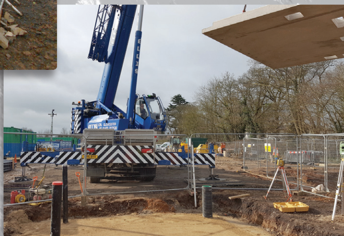
Installation of precast concrete kiosk base Courtesy of NMCNomenca
